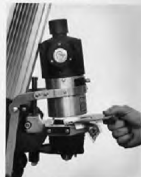
26 | replace the negative carrier
